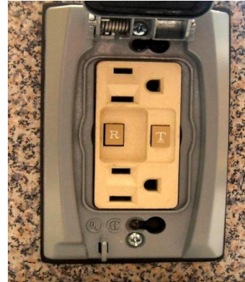
and supplies AC to the ground fault duplex.
