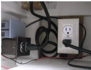
Black duplex outlet (on left) is AC from the generator
