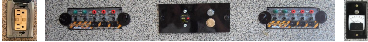
AC GF Hobby King strip DC breaker panel Hobby King strip DC Meter
