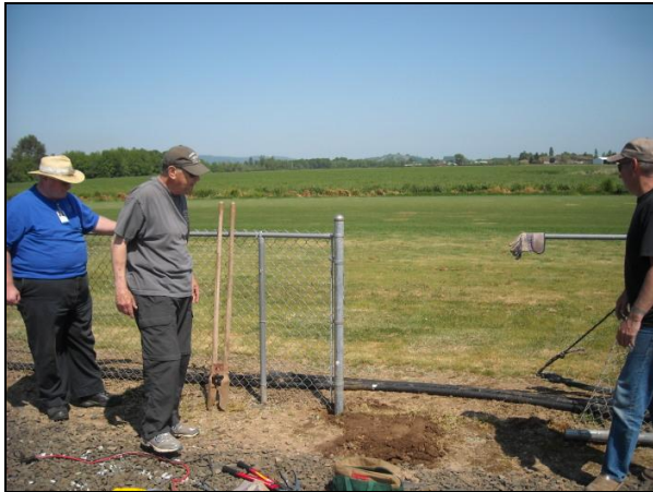
Gate post installed
