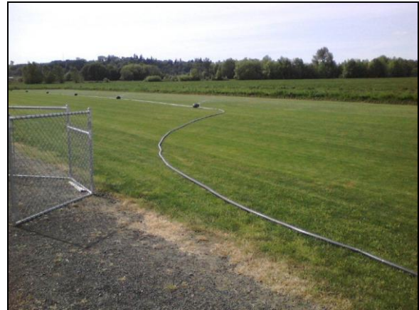
Sprinklers being tested
