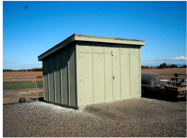
Completed and painted.
