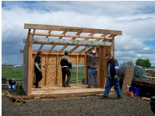
Mower shed under construction.
