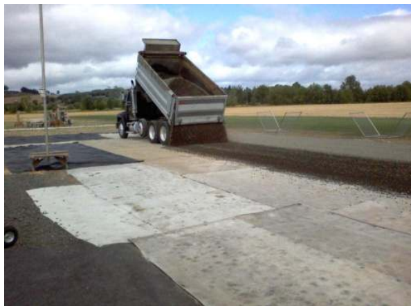
Pit area covered with 3/4 minus.
